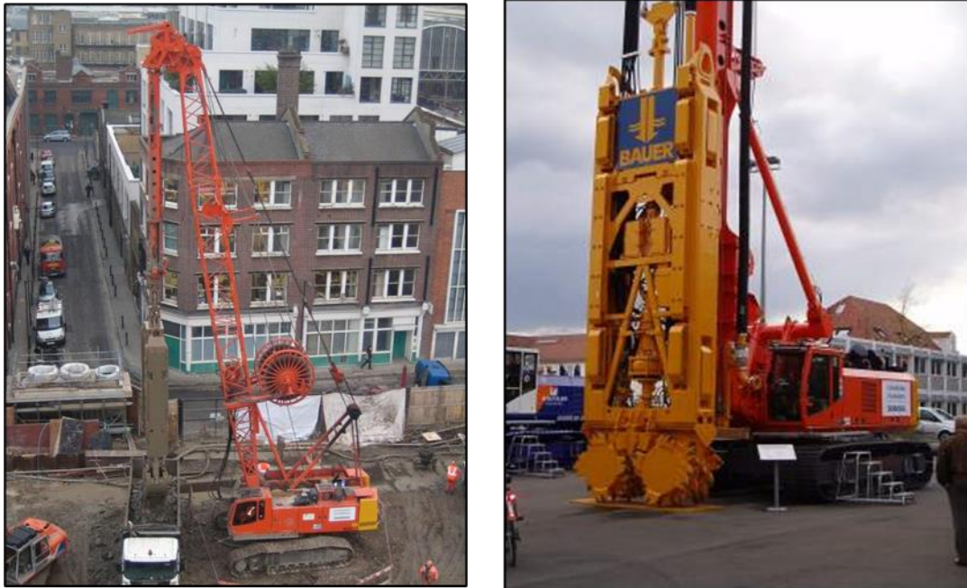
Figure 2-2: Example Photos of a Grab and Hydrofraise
