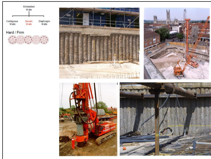
Figure 3-2: Example Secant Piling Works and Rigs
