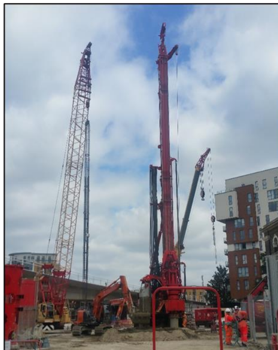
Figure 3-4: Typical Secant Pile Operation
