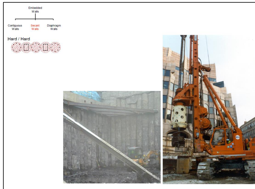
Figure 3-3: Example Secant Piling Works and Rigs
