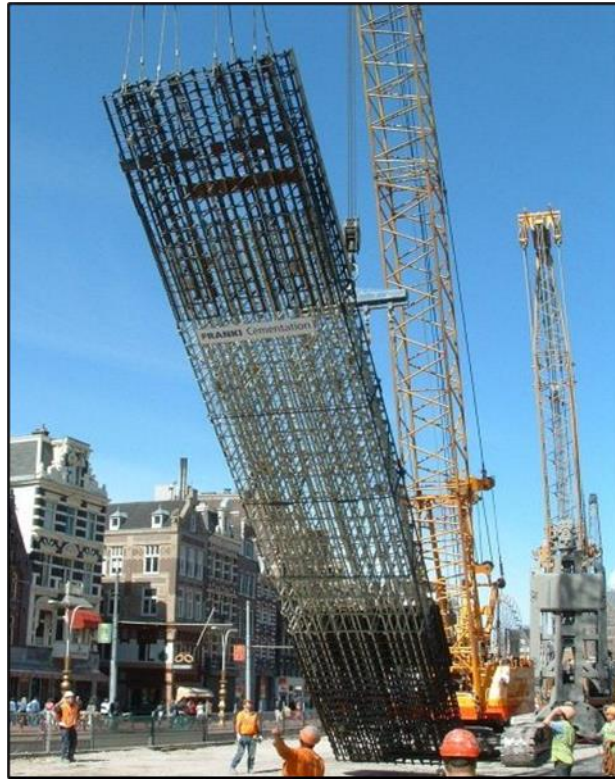
Figure 2-3: Typical Reinforcement Cage for a D-wall Panel
